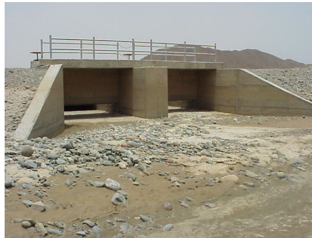
Figure 4.12 The Sheeb-Kethin culvert
