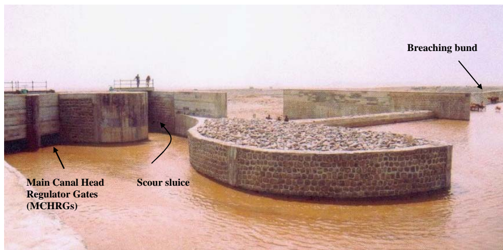
Figure 4.10 The Wadi Laba modern headwork
