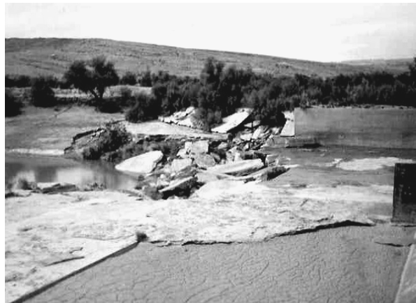
Figure 5.3 Deliberately destroyed weir in Anambar Plain, Pakistan (van Steenberg, 1997)
